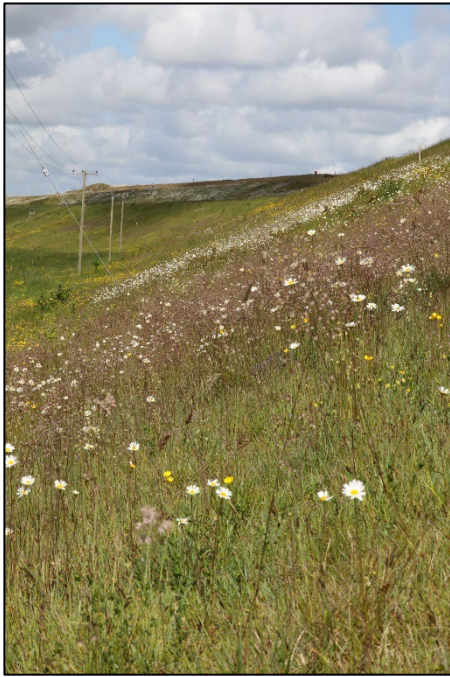
Figure 6: Photograph of embankment slope in summer
